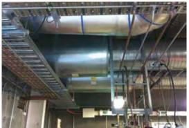
Our Industrial Cylindrical Attenuators are similar to HVAC Cylindrical Attenuators, but with heavier construction for increased durability in harsh, high noise level and exterior environments.
