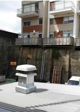
Our Curb Rectangular Attenuators are NCS/NCT/NSM/ NTM rectangular attenuators, of square dimension to suit roof fan cowl base sizes, and incorporate an extended case to provide a spacer for improved airflow and motor clearance. Specifically designed for roof penetration situations.
